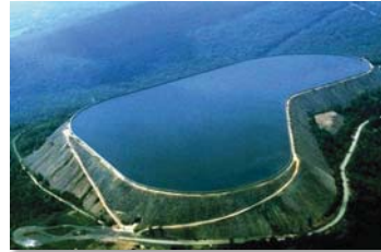
Pumped Hydro (Taum Sauk) 400 MW
