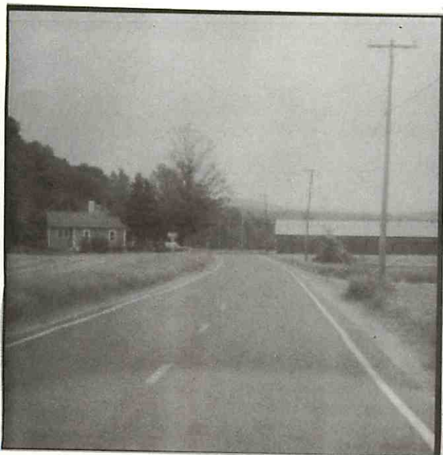
Figure 4. Road scene with other man-made structures.
