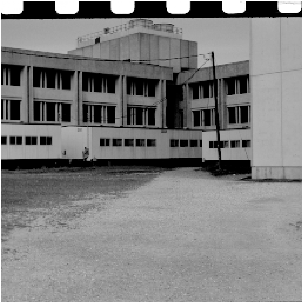
Figure 6.16: Another image of the Lederle Graduate Research Center (LGRC). Not only do the images of the LGRC view the building from different angles and at different scales, they also image different parts of building.
