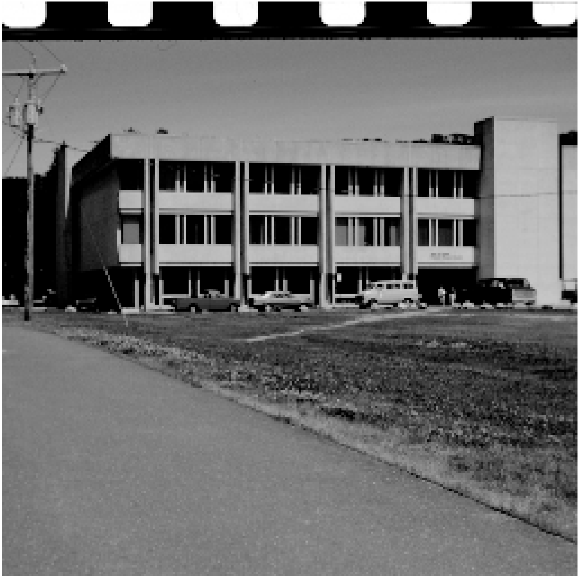
Figure 6.15: One of ten images of the Lederle Graduate Research Center (LGRC). The images were taken from random positions in the courtyard behind the building.
