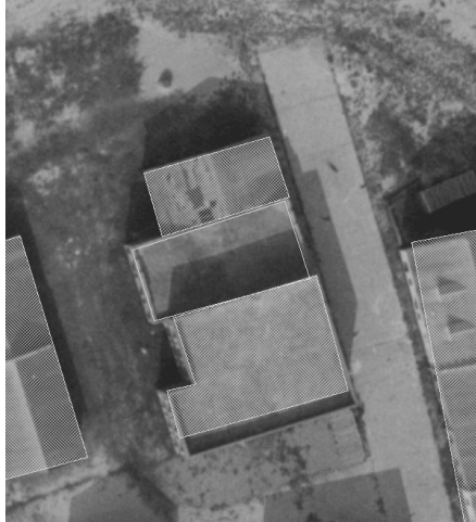
Figure 4.21. The shadow on the flat roof of this building makes a strong evidence for a center line and the roof top was misclassified as a peaked roof building.
